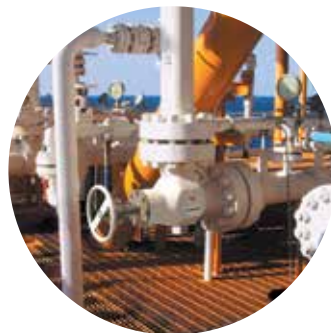
8" / ASME 1500 Angle Choke Valve
