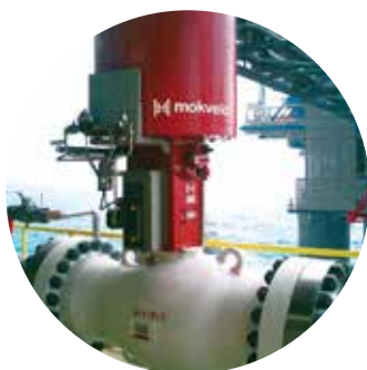
24" / ASME 1500 Axial Control Valve
