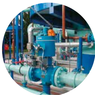
8" / ASME 600 Axial Control Valve
