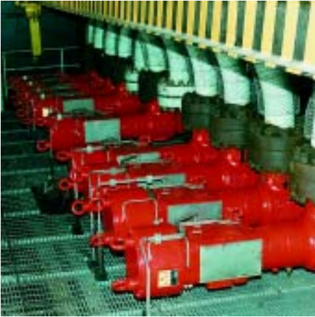
adjustable choke valves 8" ANSI 900 lbs with pneumatic actuators, gas production offshore Malaysia
