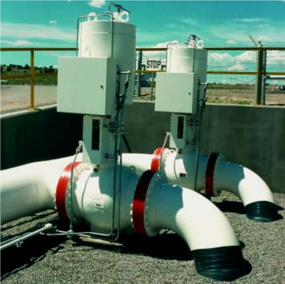
adjustable choke valves 8" ANSI 900 lbs with pneumatic actuators, gas production offshore Malaysia
